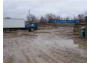
BEFORE: East end of the Recycle Center building
