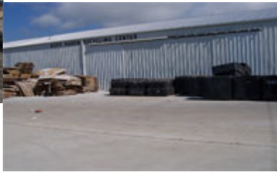
AFTER: Completed concrete driveway & storage area
