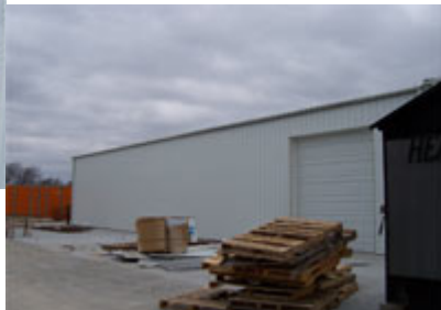
AFTER: Exterior of the completed new extension on the south side
