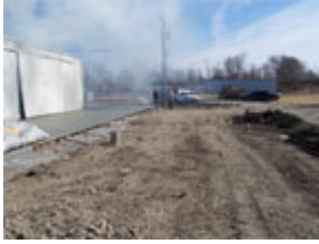
BEFORE: Southeast end; mud/gravel driveway & future storage area
