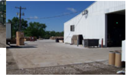
AFTER: Concrete on east end of the Recycle Center building completed
