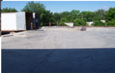
AFTER: The concrete for the dock area completed
