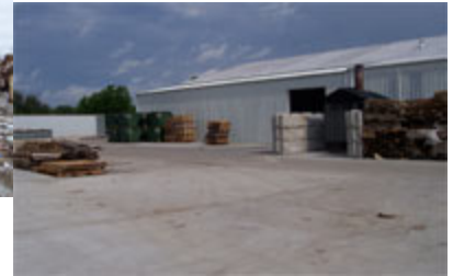
AFTER: Concrete drive & storage area
