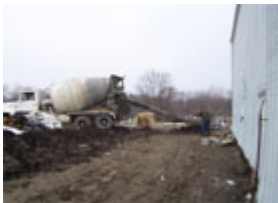
BEFORE: Exterior of the south side
